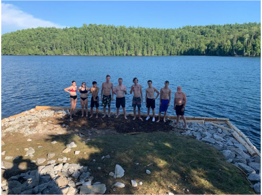
The rebuilt shoreline in front of the Jolly Roger Lodge
