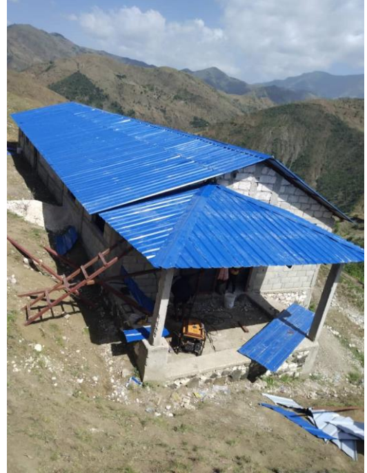
The new roof installed on Bonplan Methodist Church, September 2023
